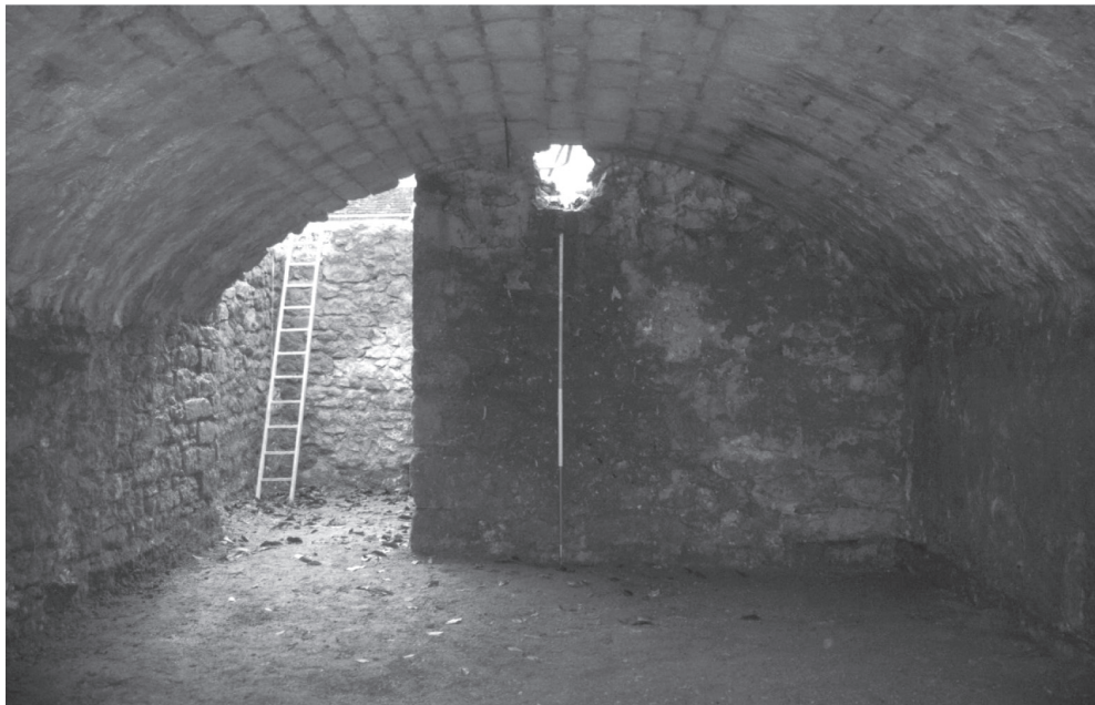
Fig. 8. Barrel-vaulted cellar 433 at ground level showing fireplace 432, looking south (above); interior of barrel-vaulted cellar 433 showing stairwell, looking south (below).
